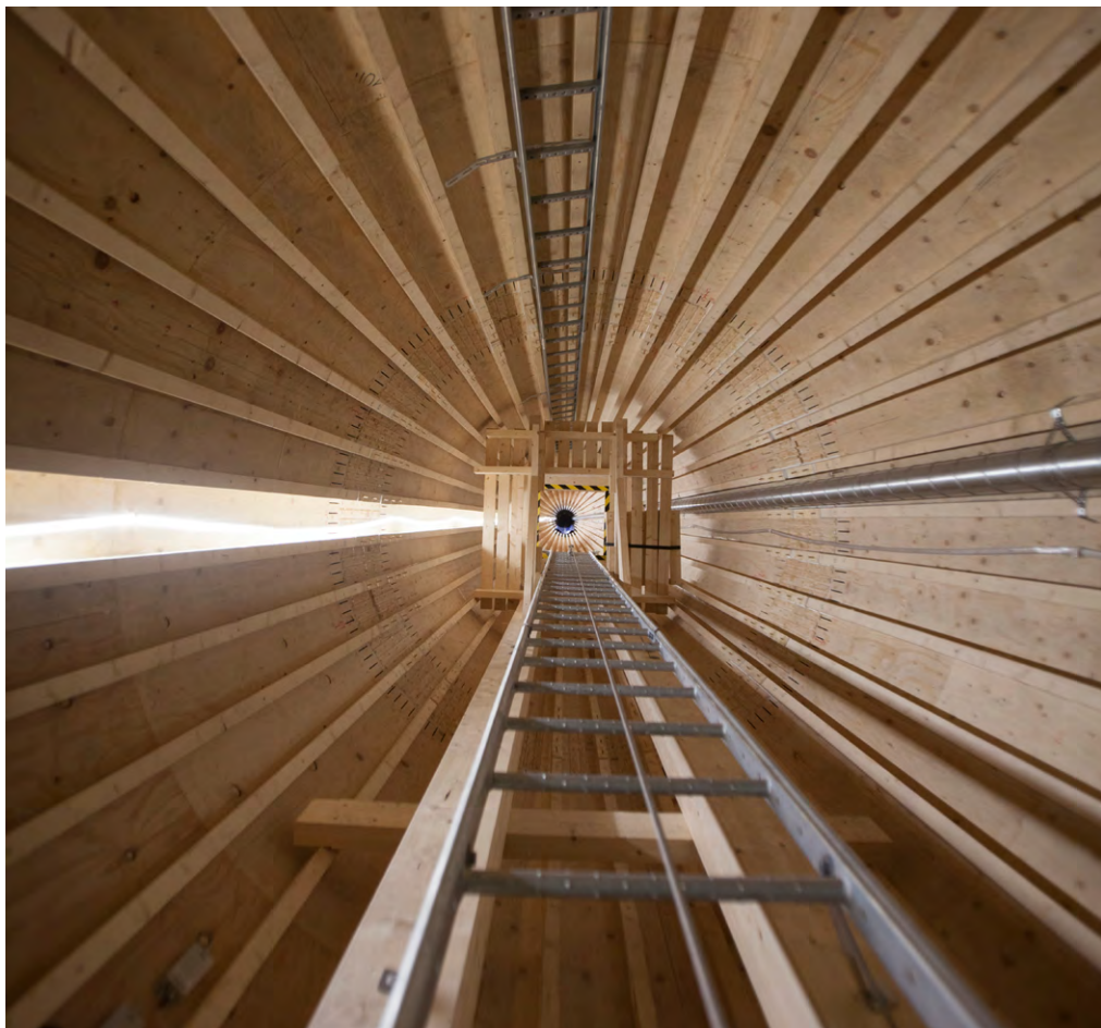
← View from inside of the first Modvion™ wooden prototype tower. The 30 meter tower is installed in the archipelago by Gothenburg, Sweden.
